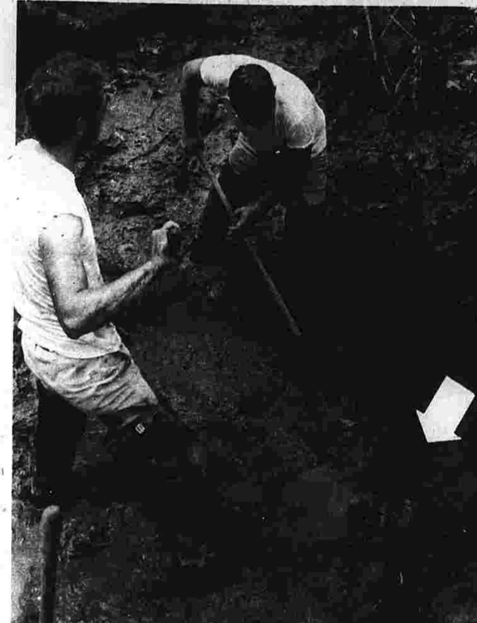
Town of Manchester Public Works personnel work to uncover the ruptured wooden pipeline, indicated by the arrow. The pipe line was shattered Wednesday morning when a bulldozer ran over a boulder, forcing it down through four feet of soft ground, smashing the pipe. The metal spiral visible in the mire was a part of the wooden pipeline, which was made up of planks, wrapped tightly with wires. By about 3 p.m. the repair crew had the damaged section of pipeline uncovered. (Herald photo by Knapp)
